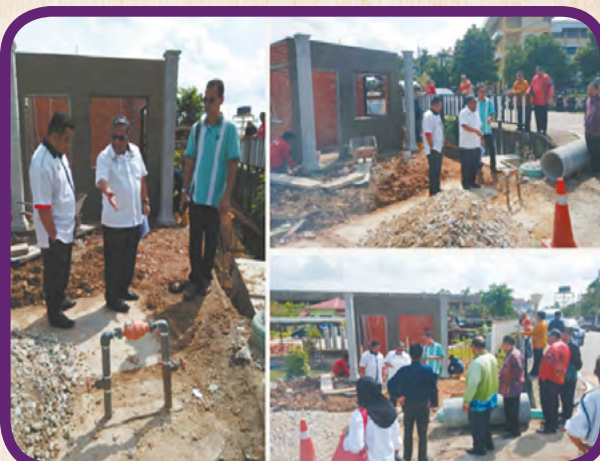
Repairing school fences at SMK Durian Daun, Melaka
