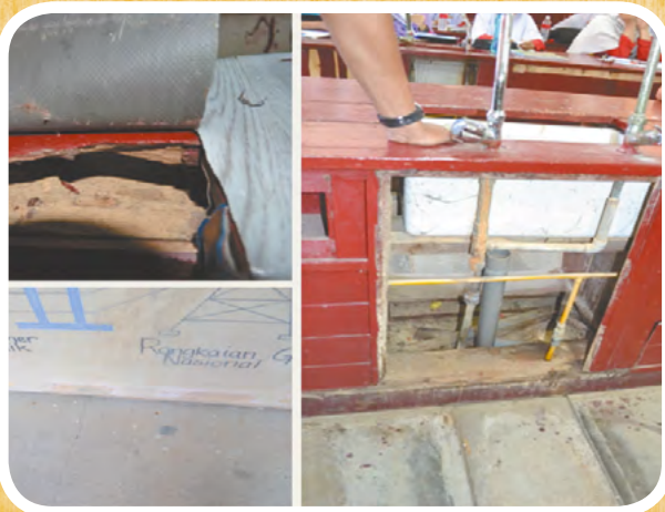
Termite Control at SMK Dato' Mahmud Paduka Raja (1)
