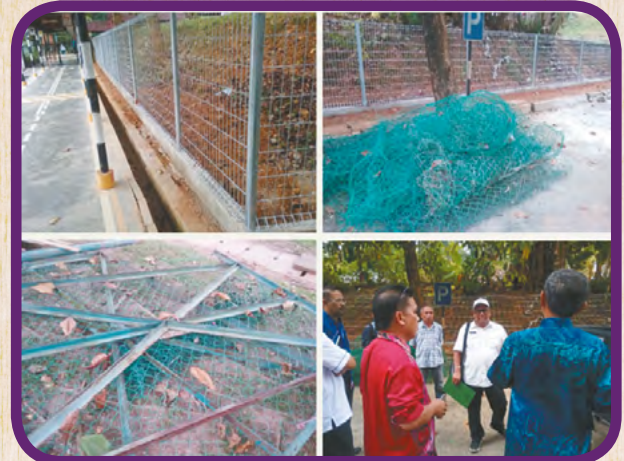
Repairing school fences at SMK Taman Bunga Raya, Rawang
