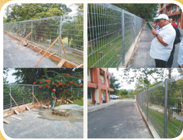
Repairing school fences at SK Sungai Buaya, Rawang
