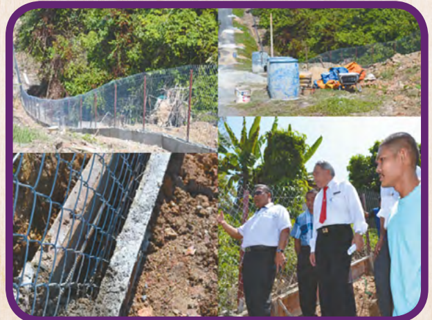
Repairing school fences SMK Tengku Ibrahim, Terengganu
